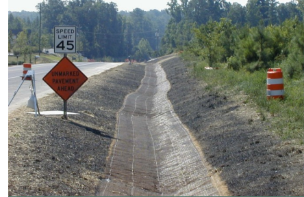
Phase 1 Unvegetated channel protection
