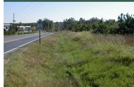
Phase 3 Permanently reinforced turf
