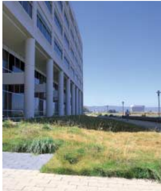
Fire lane, San Mateo, CA—Many native grasses and other attractive vegetation can be grown in Grasspave 2 .
