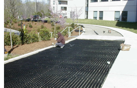
Grasspave 2 system rolled into place
